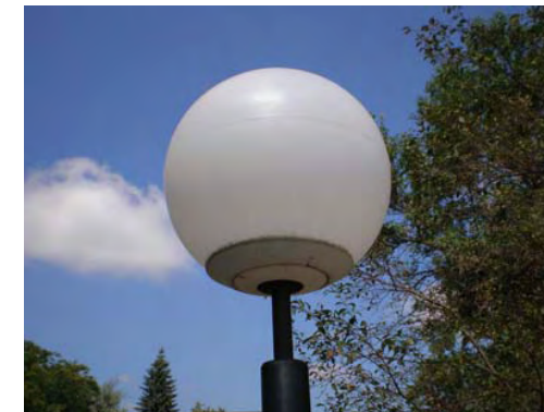
Lighting along Sidewalk
